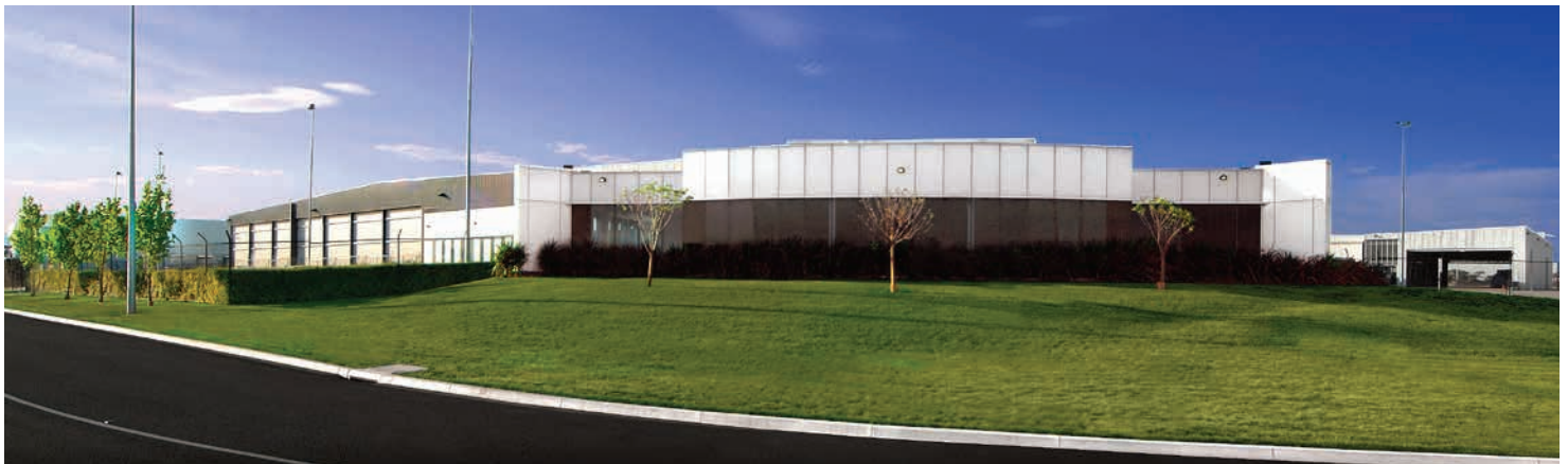
Austrak Business Park, Somerton, VIC
