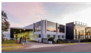
21-23 Wirraway Drive, Port Melbourne
