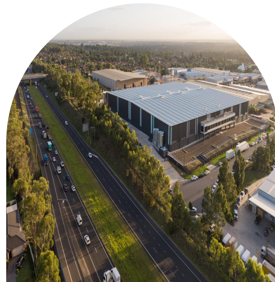
42 Cox Place, Glendenning, NSW
