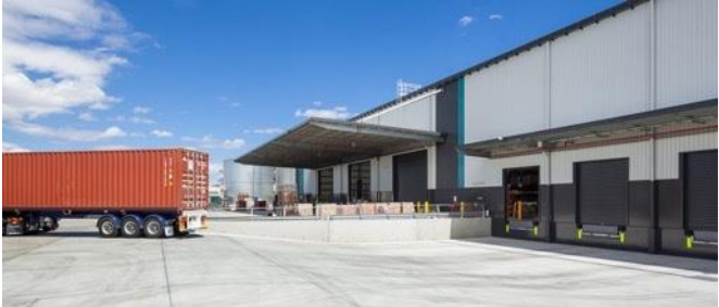
Seven Hills, NSW 1 Re-leased facility at market rents
