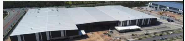
2020 Underway Developments 4 facilities totaling $167m
