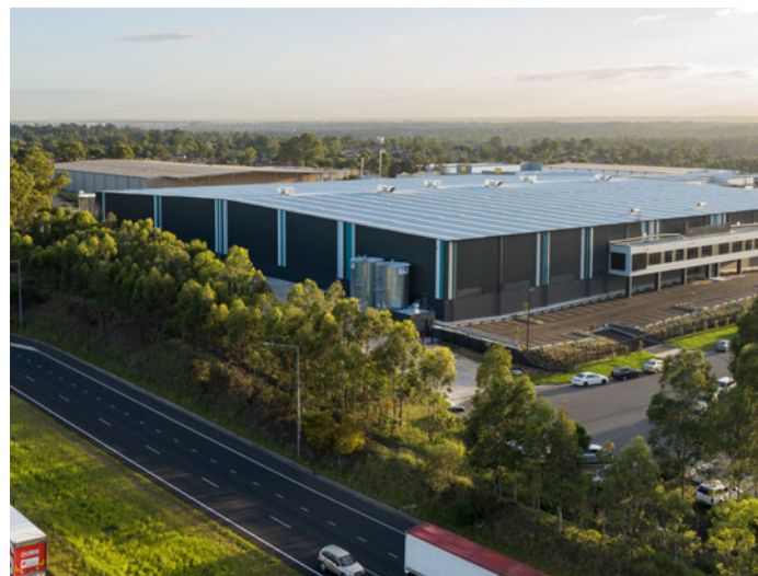
42 Cox Place, Glendenning, NSW
